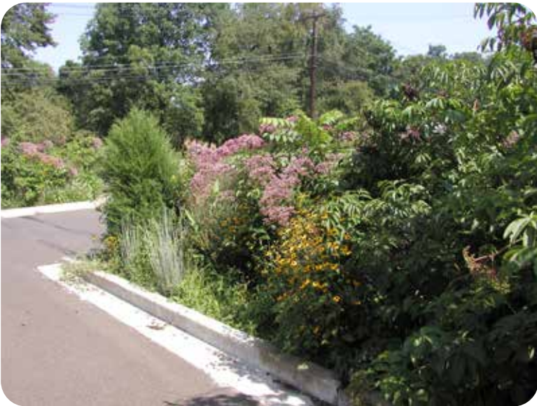
ENHANCED STORMWATER MANAGEMENT FEATURE, GWYNEDD MERCY COLLEGE.
