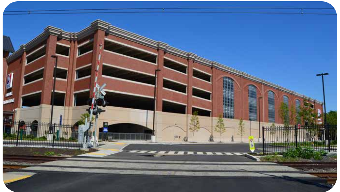
SEPTA LANSDALE STATION GARAGE OPENED IN 2017.
