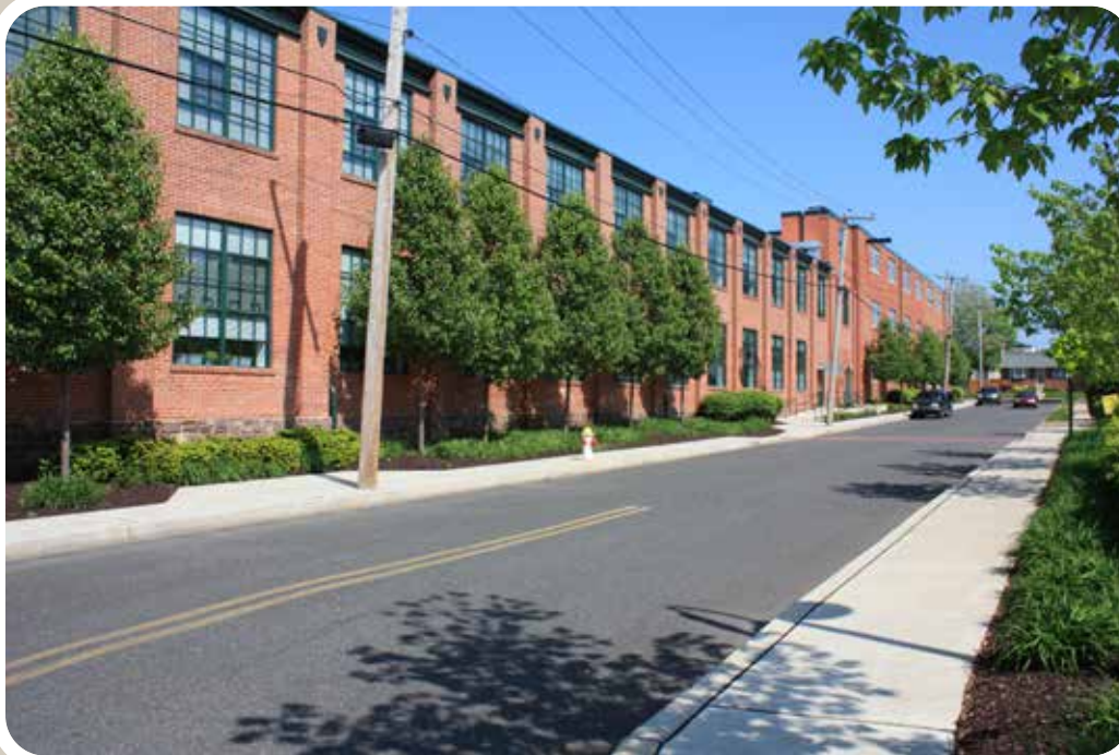
#39 ON THE HISTORIC RESOURCES TABLE/MAP IS THE HISTORIC DEXDALE HOSEIERY MILL (NOW THE “TURBO LOFTS”).
