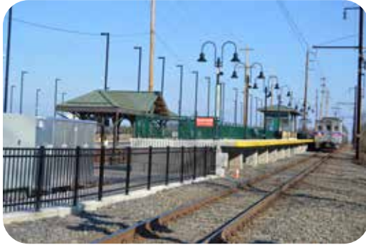
LANSDALE'S 9 TH STREET STATION IS THE NEWEST STATION IN SEPTA'S REGIONAL RAIL SYSTEM.
