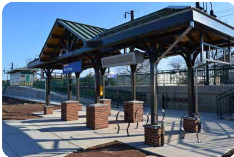
THE BICYCLE SHELTER AT NINTH STREET STATION ENCOURAGES TRANSIT RIDERS TO BIKE, RATHER THAN DRIVE TO THE STATION.
