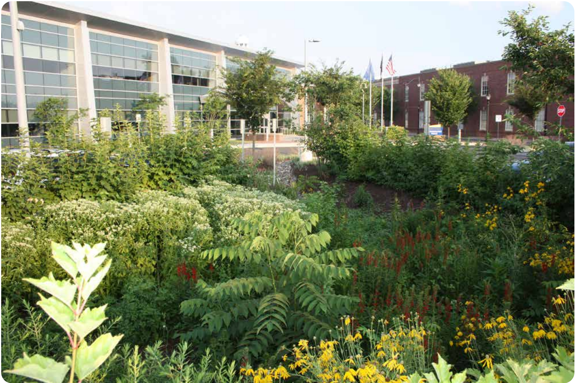
THE RAIN GARDEN IN THE PARKING LOT OF LANSDALE'S MUNICIPAL COMPLEX FILTERS POLLUTANTS AND SUPPORTS STORMWATER INFILTRATION.
