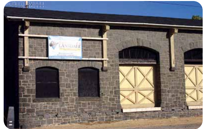
THE FREIGHT STATION, LOCATED ACROSS THE STREET FROM BOROUGH HALL, REPRESENTS AN EXCELLENT ADAPTIVE REUSE OPPORTUNITY.
