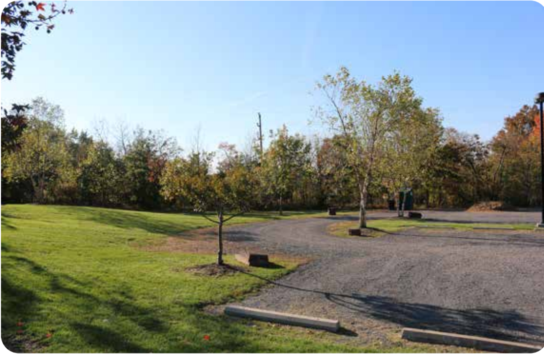
STONY CREEK PARK'S LOW-IMPACT PARKING LOT IS DESIGNED TO DETAIN AND INFILTRATE STORMWATER.
