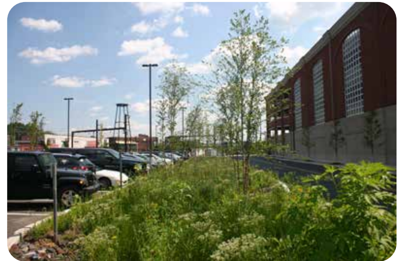
THE SEPTA GARAGE AT LANSDALE STATION INTEGRATES STORMWATER MANAGEMENT BEST PRACTICES WITHIN ITS SURFACE PARKING AREA.
