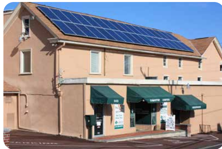
SOLAR PANELS ON THE ROOF OF A SMALL BUSINESS IN HARLEYSVILLE.
