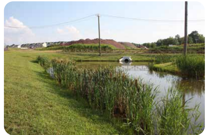
THE RETENTION BASIN BEHIND THE ANDALE GREEN TOWNHOUSE DEVELOPMENT CAPTURES, CONTROLS AND FILTERS STORMWATER RUNOFF.
