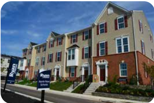
WILLIAMSON SQUARE AND ANDALE GREEN TOWNHOMES WERE ALL CONSTRUCTED IN RECENT YEARS.
