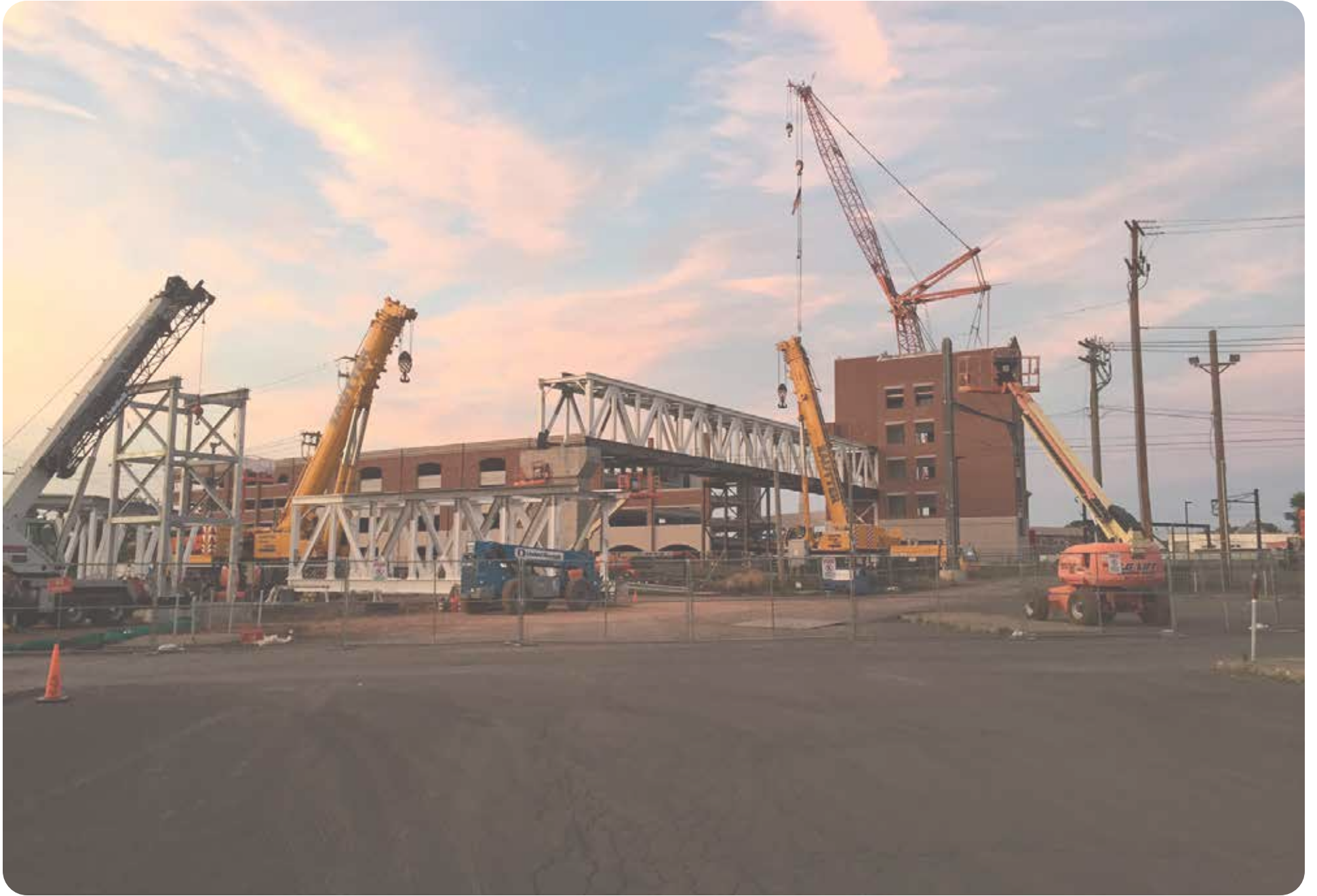
RECENT CONSTRUCTION OF LANSDALE SEPTA GARAGE AND PEDESTRIAN BRIDGE.
