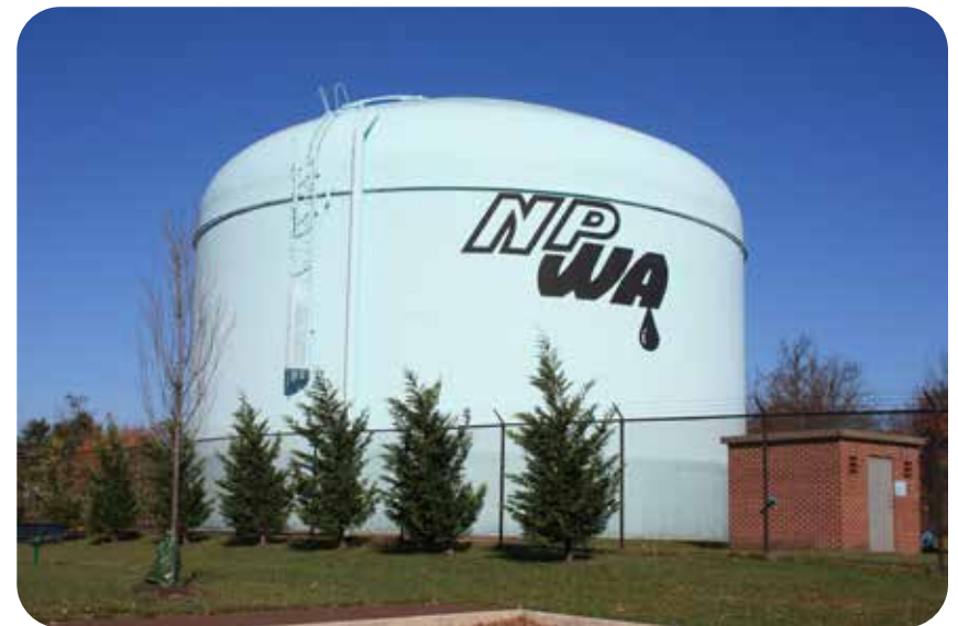
THE NORTH PENN WATER TANK NEAR FREDERICK AND CLEAR SPRING ROADS IS SCHEDULED TO BE REPLACED IN THE NEAR FUTURE. THE NEW TANK WILL BETTER HELP THE AUTHORITY MEET MORE STRINGENT WATER QUALITY STANDARDS.
