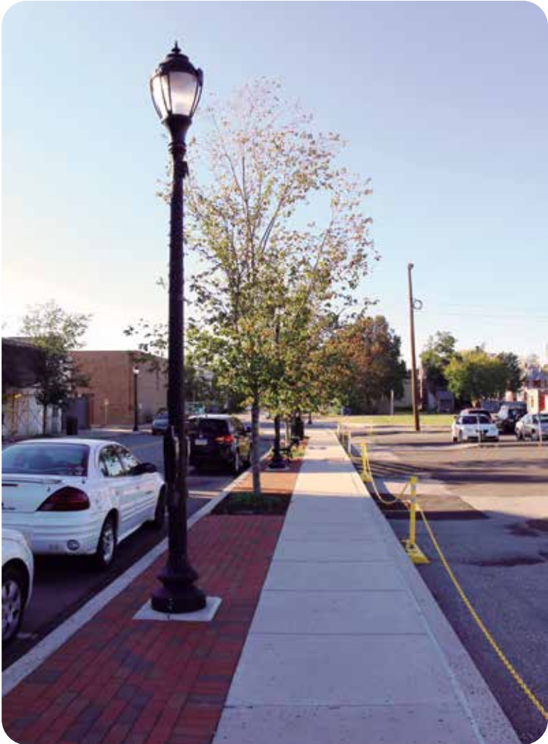
THE BOROUGH PARTICIPATES IN DVRPC'S REGIONAL STREETLIGHT PROCUREMENT PROGRAM, LEADING TO ENERGY AND COST SAVINGS.
