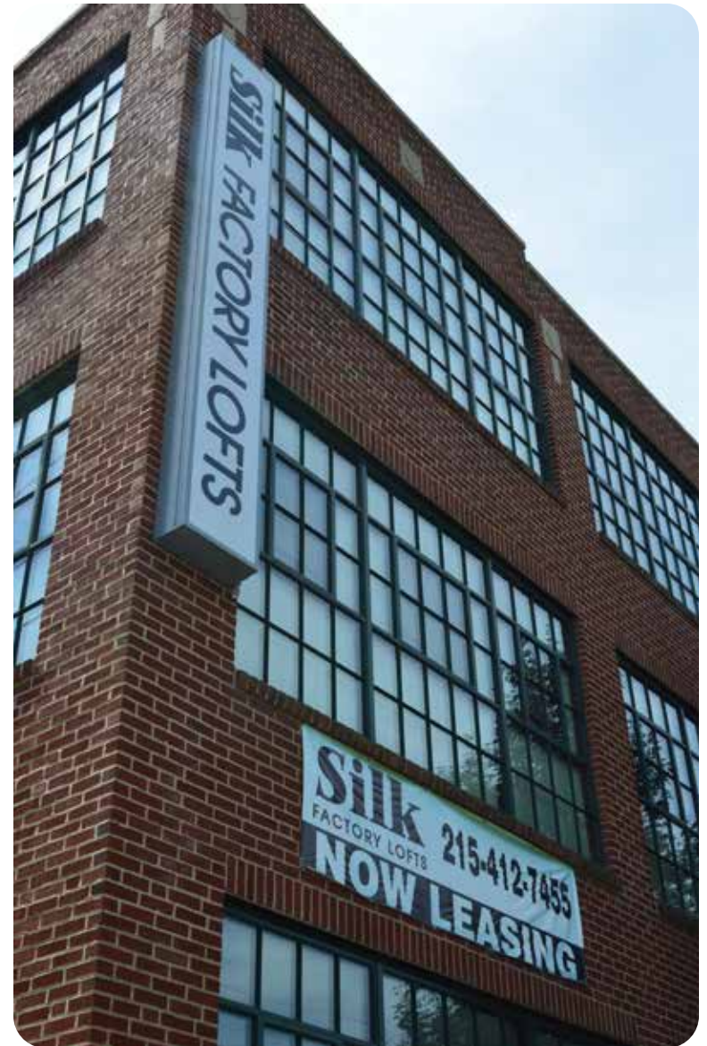
REDEVELOPMENT OF THE FORMER INTERSTATE HOSIERY MILL AND SANTAERIAN DEPARTMENT STORE AS THE SILK FACTORY LOFTS ADDED A STYLISH RESIDENTIAL COMMUNITY TO THE BOROUGH.
