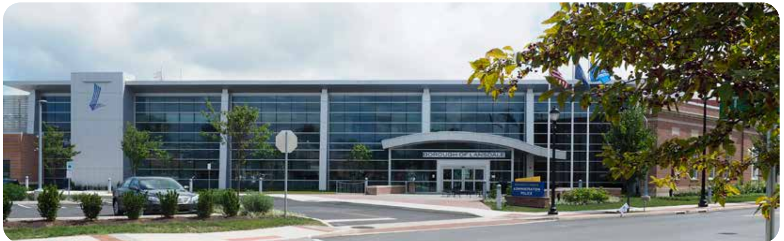
THE LANSDALE MUNICIPAL COMPLEX WAS AWARDED LEED SILVER CERTIFICATION.
